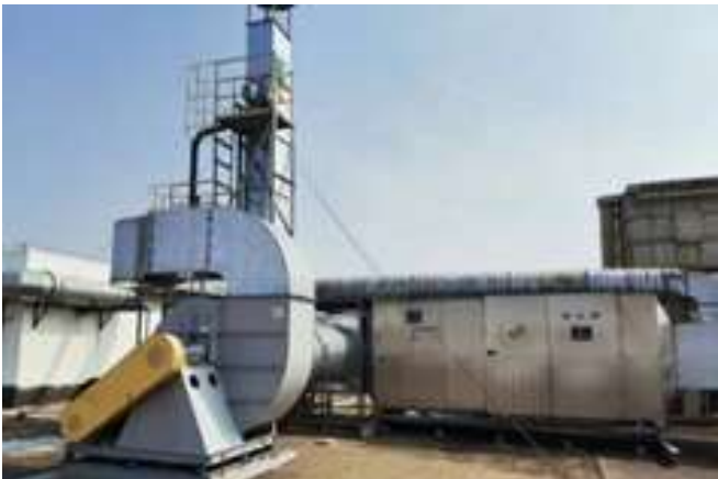
Organic waste gas treatment equipment: UV+ activated carbon equipment
